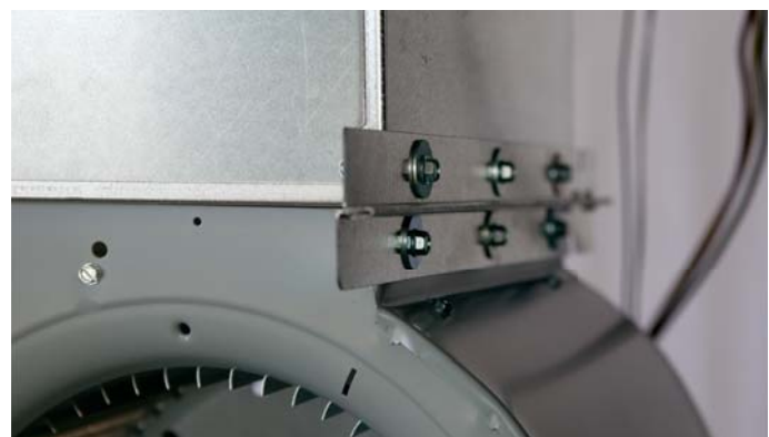
Figure 2: Blower Housing Connections
